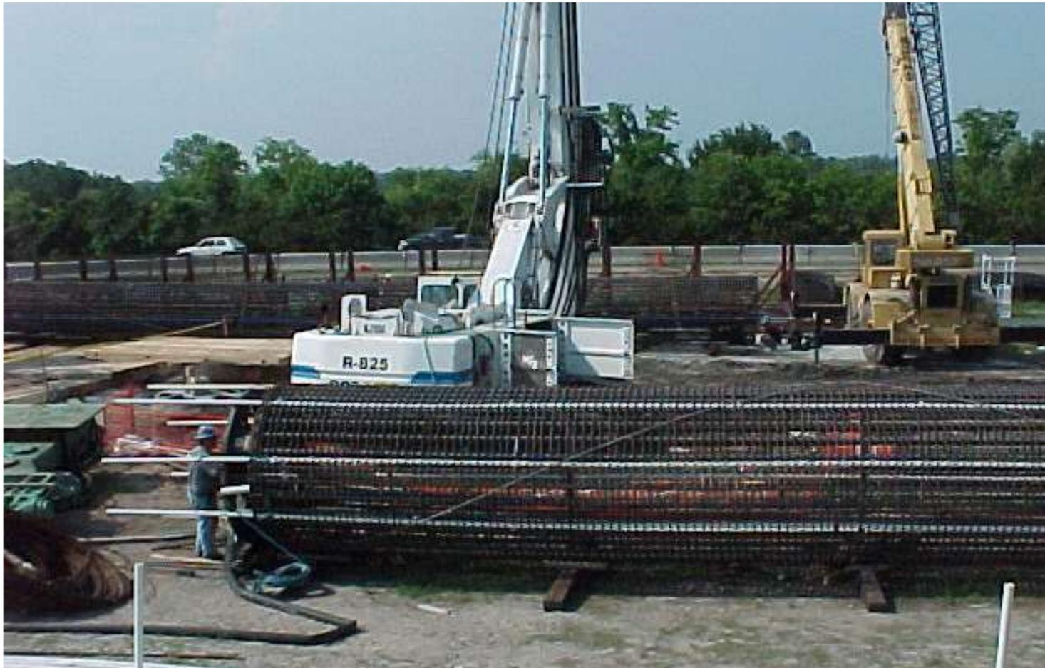
**Deep Foundations: 2.5 m- and 3-m diameter drilled shafts with lengths of 45 to 60 m**
